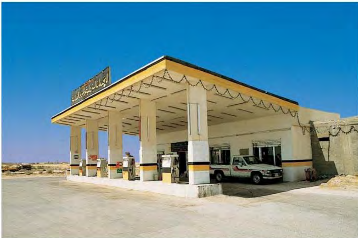
A petrol and services station in Raghbah
