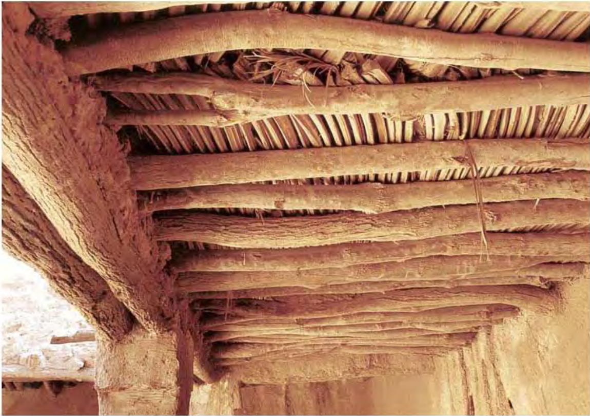
Roofing style of houses
