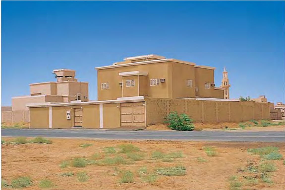
A typical modern house in Raghbah
