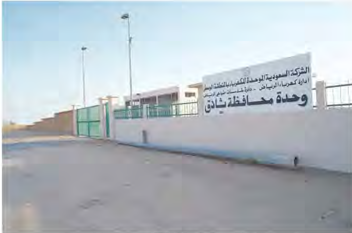
Thadeq Power Plant
