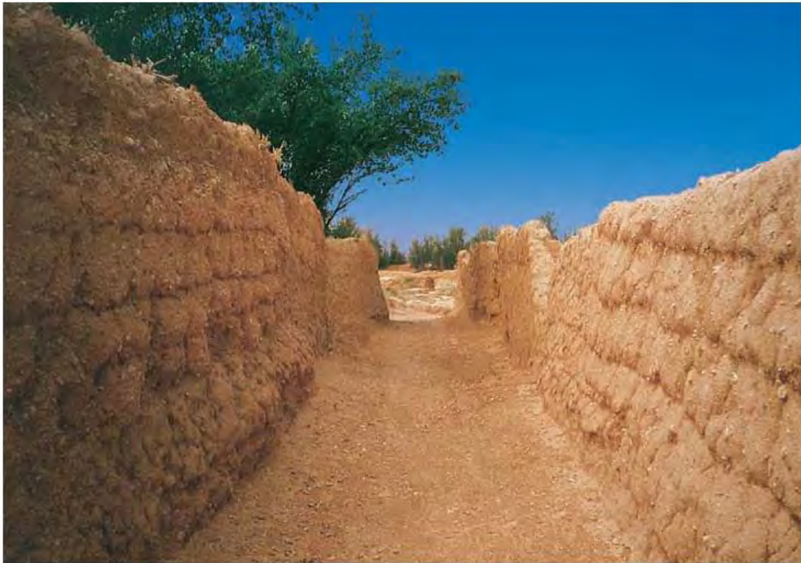
Pattern of building with mud layers
